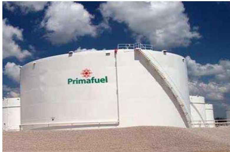
Gambar 2. 2 Floating Roof Tanks .
